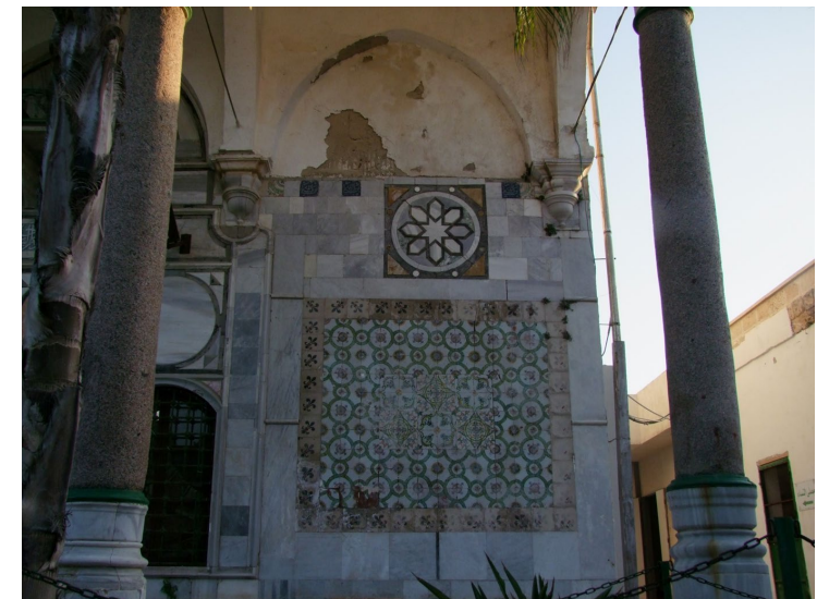
The weathering in the marble and qashan inlay, in the western corner, along the facade of the prayer hall (the arcade)
